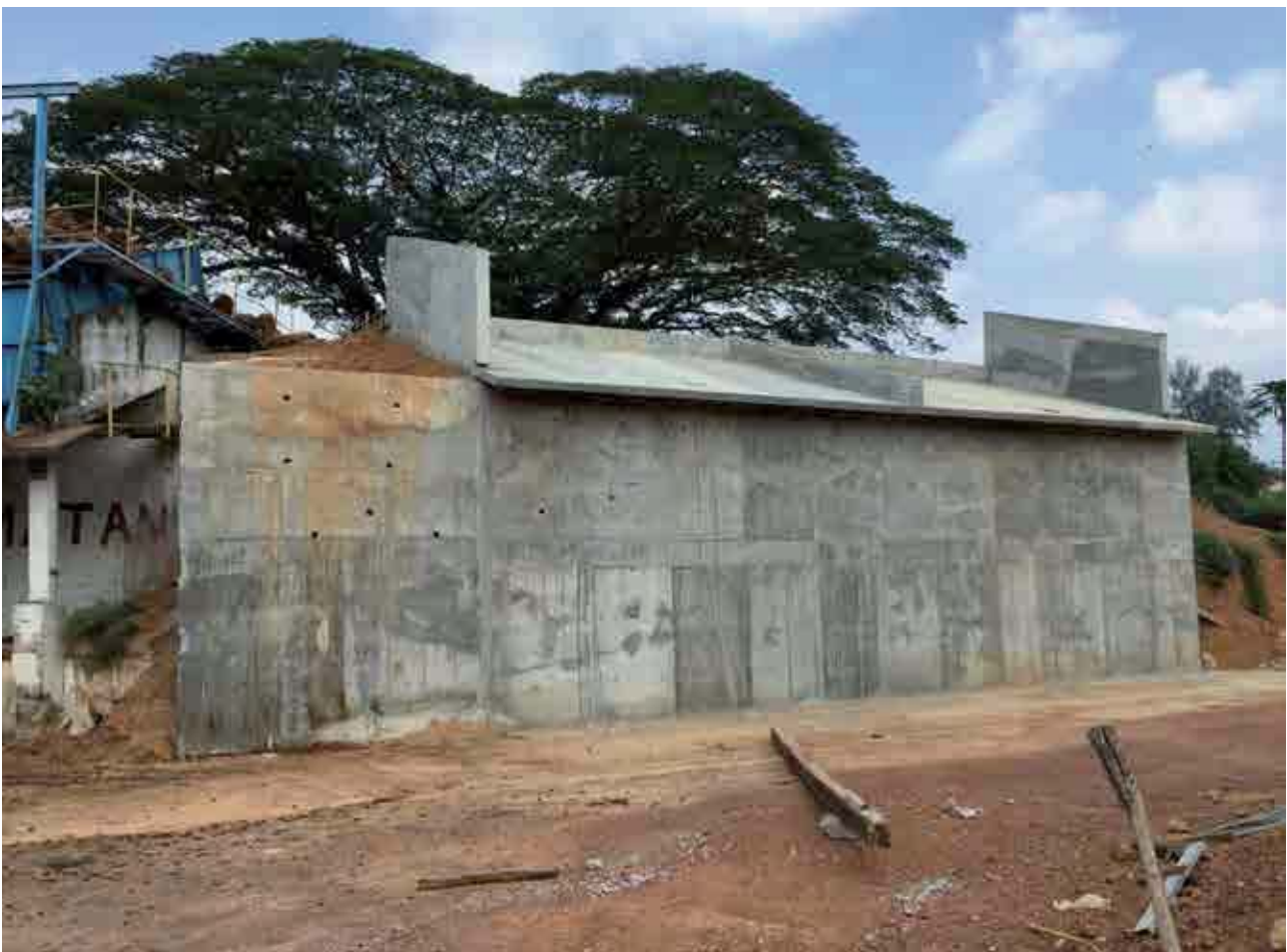
Ramp : New Ramp being constructed at Buloh Akar Estate
